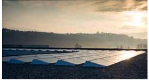
ture of this unit is the T10 support structure, an innovative technology that guarantees stability and yet avoids drilling holes or using ballast, and does not affect the roof's sealing integrity. It can withstand winds of up to 190 kilometers per hour, and is robust enough to weather a tornado.
