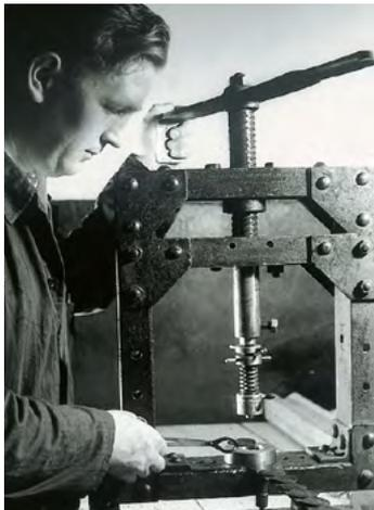
First seals produced on a spindle press, 1929
