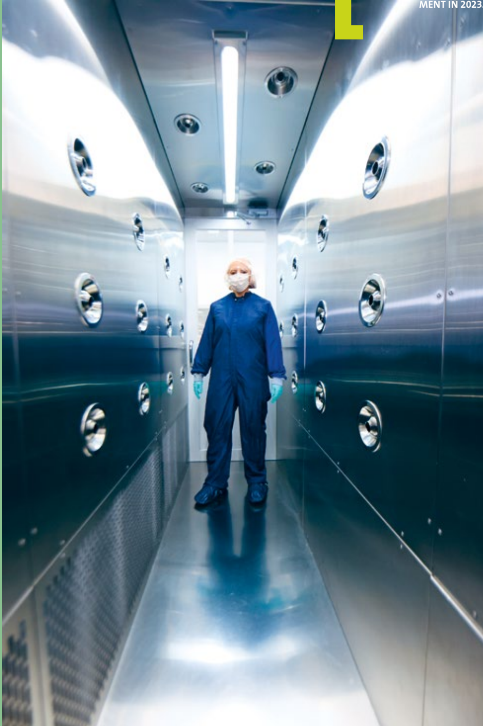
Battery systems – Midland, USA The airlock connects the changing room with the battery cell production facility. Nozzles blast air from all sides for 15 seconds, removing any dust particles from protective clothing. Then the airlock door re-opens and the cleanroom can be entered.
